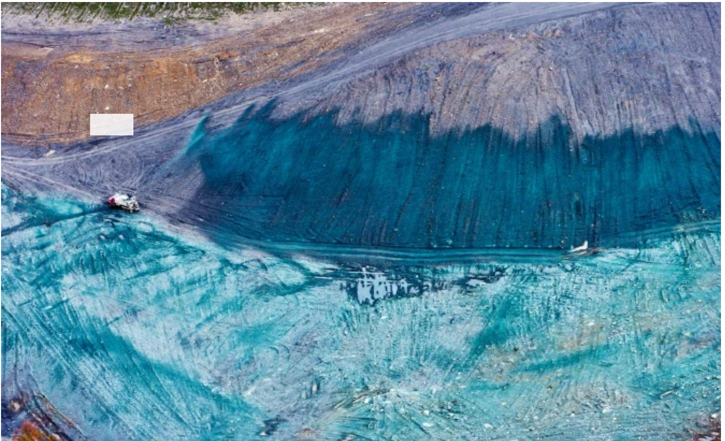
Hydro-seeding. Grass being planted on covered Mountaintop Removal mining site around Kayford Mountain, WV
